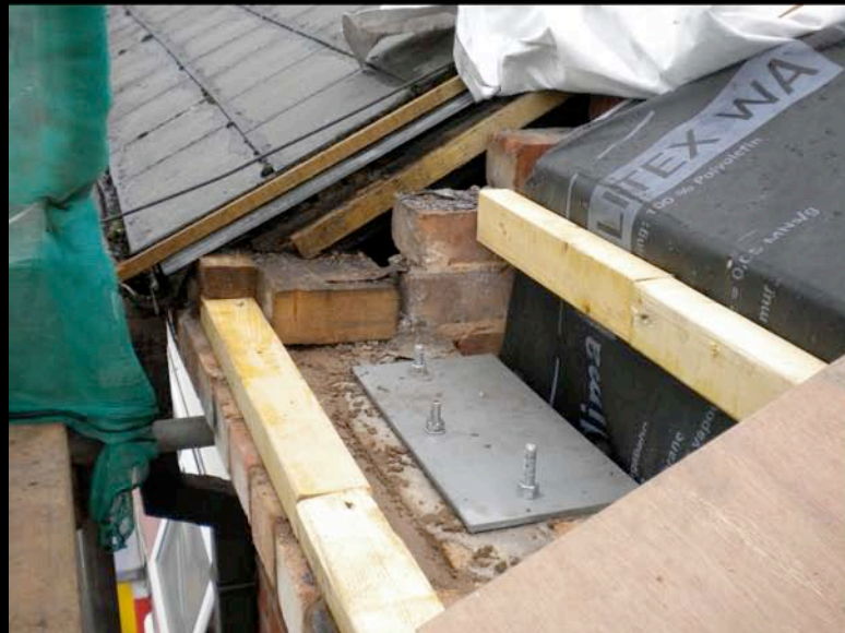
Roof pod footing to terrace walls.
